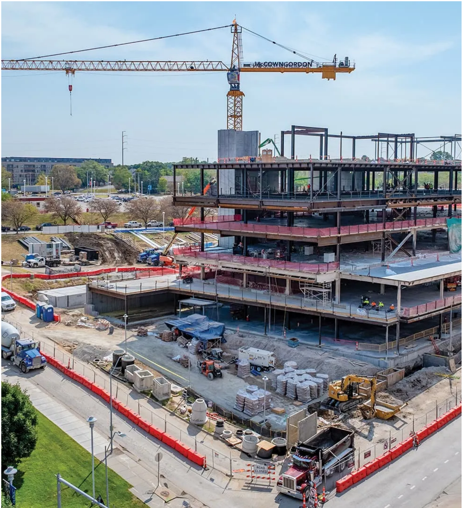
Healthcare Delivery and Innovation Building construction site on Sept. 17, 2025.
